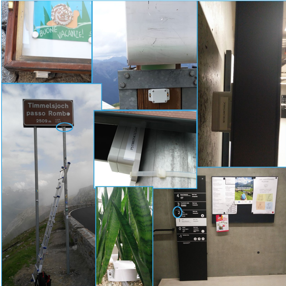
Figure 2: some examples of installations.
